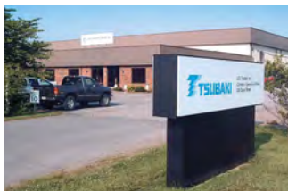
UST Portland Plant
