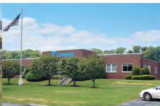
UST Holyoke Plant
