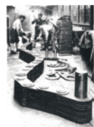
Assembling a chain for use in floodgates (around 1930)
