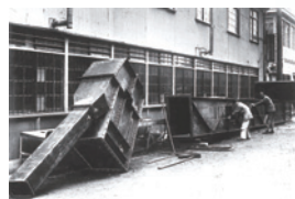
Part of the first large-scale conveyor plant delivered by the Company (1937)
