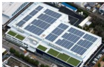
The solar power generation system of the new materials handling systems factory
