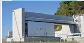
Floodgates Cable carriers
