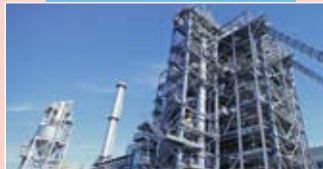
Biomass power plants Bucket elevators, conveyor chains
